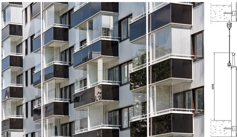
Figure 4. Example of typical balcony renovation work. The balcony slab and side wall are fixed, the balustrade varies from a concrete parapet to a glass-aluminum balustrade with balcony glazing installed (pictures courtesy of Lumon Oy).
