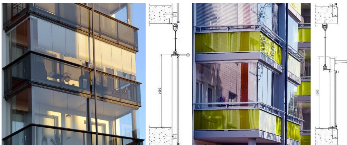
Figure 1. Two examples of the most typical balcony, balustrade and balcony glazing solutions currently in use in Finland in new constructions (pictures courtesy of Lumon Oy). The commonly used balcony glazing blinds [12] are shown in the left picture.
