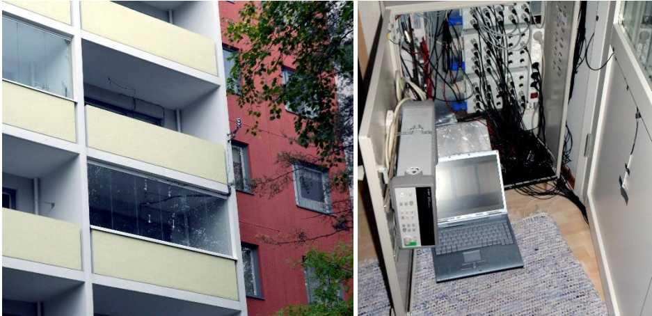
Figure 14. South-western façade of the building F (left) and the measuring equipment (right).
