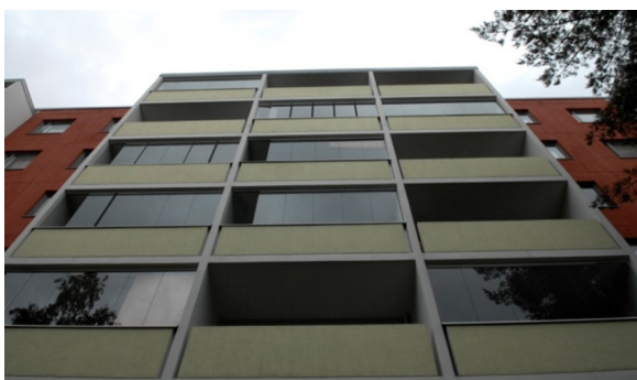
Fig. 2. Balconies with openable balcony glazing in a 1970s apartment building.
