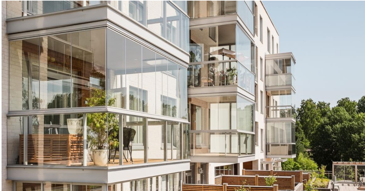
This photo depicts a Lumon balcony enclosure that matches the type used for this example modelling application. Only the operable glazing units have air spaces between each unit – the lower fixed glazing is effectively sealed and continuous.
