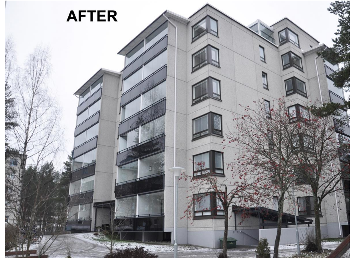
The retrofit building now features an updated façade and enclosed balconies that will improve energy efficiency, comfort and durability.
